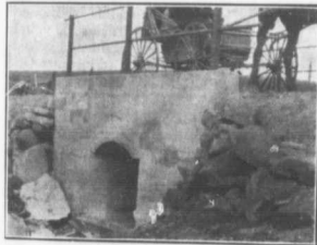
A Good Style of Road Culvert in Halton Co., Ont.
