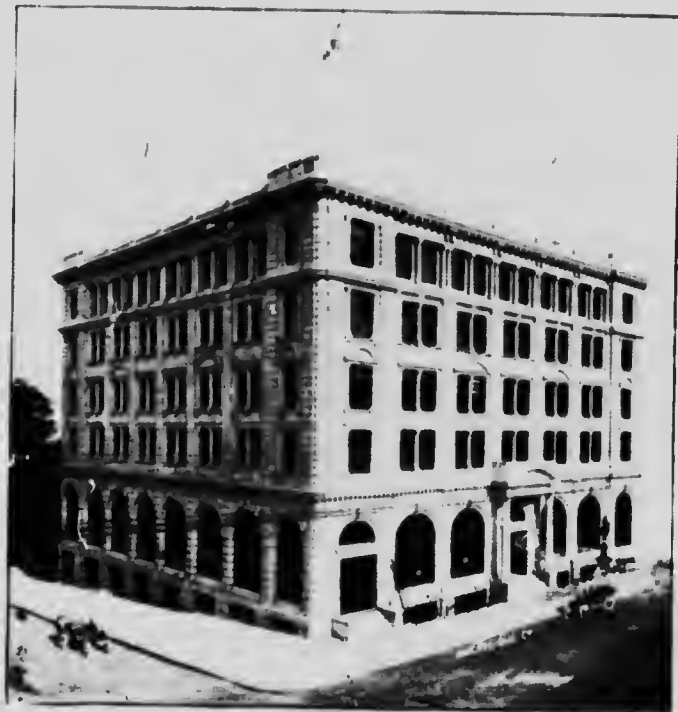
WINCH BUILDING, No. 2 ON KEY MAP
