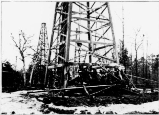
Rotary method of drilling, Caddo field, La., U.S.A.
