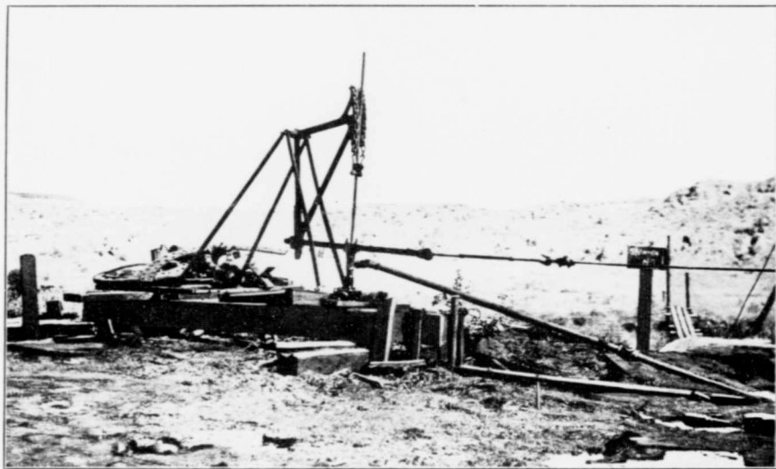
Pumping well, showing connexion with cam wheel.
