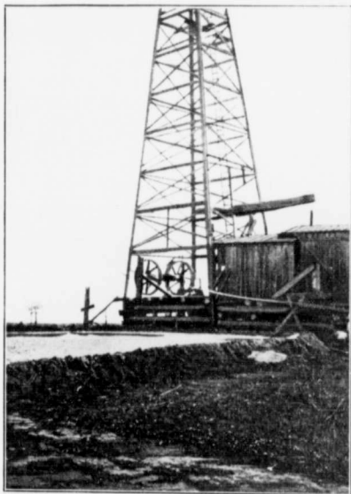
Raised derrick, showing "sludge pool," Oil City, Caddo field, La., U.S.A.
