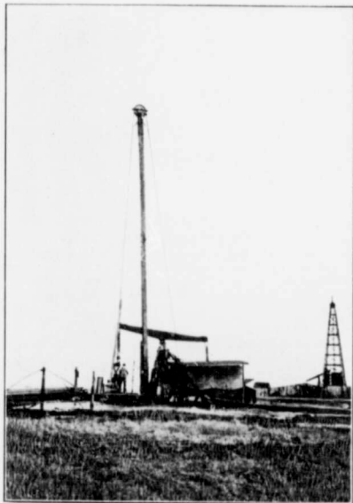
Cleaning well with Star No. 27 drilling machine, Muskagee field, Okla., U.S.A.
