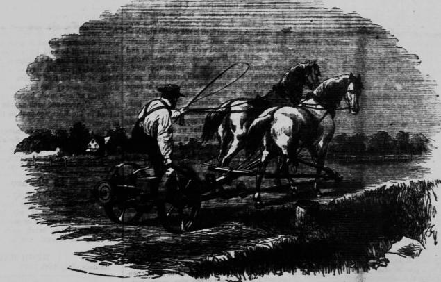
BUCKEYE MOWER WITH CUTTER BAR RAISED TO PASS AN OBSTRUCTION.
