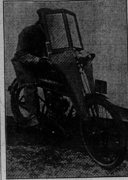
dscreen is adjustable. The aprons are designed to protect the legs from rain and mud.
