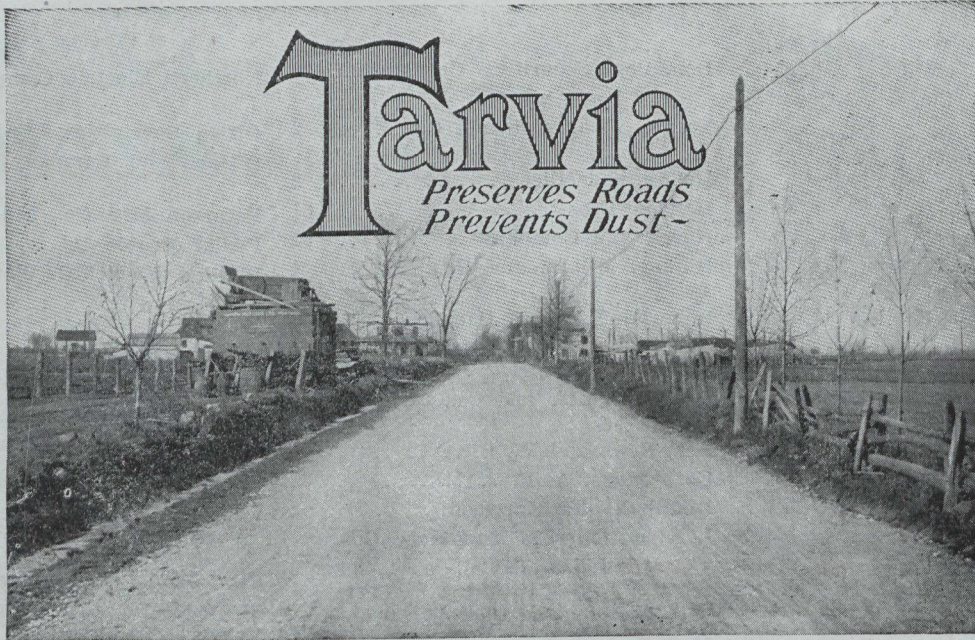
Beaconsfield Station Road, Beaconsfield, P. Q. Constructed with "Tarvia-X", Penetration Method, in 1912. Seal Coat of "Tarvia-A" applied in 1915.
