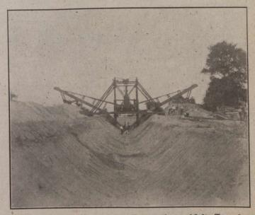
Austin Trenching Machine Excavating a 16-ft. Trench.
