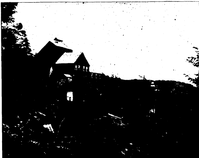
LE ROI SHAFT HOUSE, ROSSLAND.
