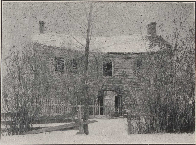
ARCHIBALD MCNEIL RESIDENCE, CLARKVILLE.
