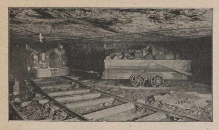
hauled. Then the trip rider uncouples the cable and drags it into that room for the car. The arrangement is such that the cable may be paid out from either end of the locomotive. Ordinarily, however, it is more convenient to take the cable out past the motorman, as that end of the locomotive is then opposite the room mouth, and the motorman can watch the light carried
