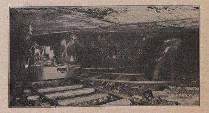
are required to make up a trip. Then it pushes them together, they are coupled up, and hauled to the partings. On the return trip the entry cars are distributed in the entry from which the loads have just been removed, and the locomotive gathers the loaded cars from the entry which was supplied with empties on the preceding trip.
