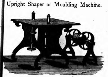
This machine is calculated to perform work that can be done by no other machine now in use, cutting straight moulding, as well as the most irregular forms. It is an indispensable machine for saving labor in railroad, carpenter and machine shops, also in agricultural and cabinet factories.
