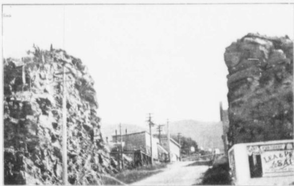
View of street cut through solid rock in a city in Western Canada. To utilize the lots facing this street the rock has to be removed from the building sites at great expense.
