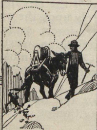
Extending Telephone Line to 9,000-Foot Level!
