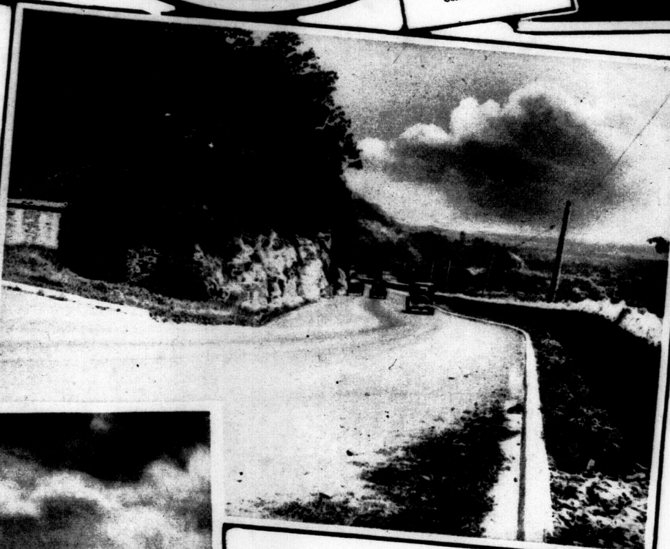
The new road up the Dundas mountain between Dundas and Bullock's corners is a stiff climb
