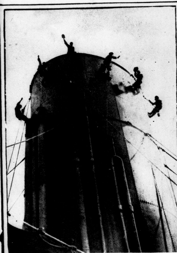
The largest funnel on any single-stack vessel, on the Atlantic liner Minnewaska. It is 24 feet in diameter and 116 feet high
