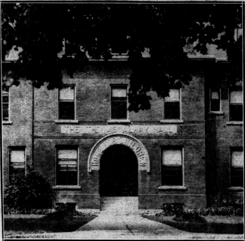
REBUILT AFTER FIRE.
