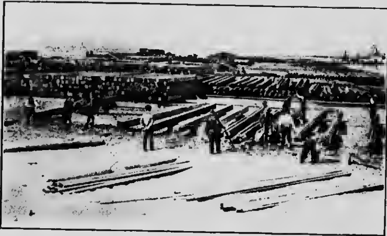
FIG. 2. — Douglas Fir Timbers for Use in Toronto, Ont., Harbor Construction.
