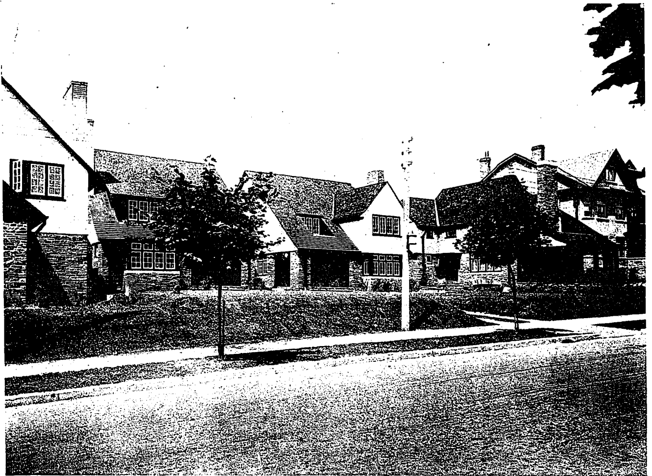
VIEW FROM STREET, LYNDHURST AVENUE DEVELOPMENT, TORONTO.
