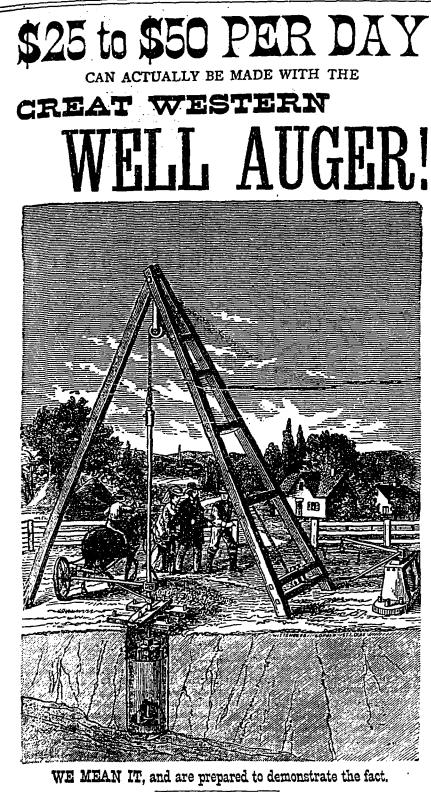
COUR AUGERS are operated entirely by HORSE POWER, and GUARANTEED to bore at the rate of 10 to 15 FEET PER HOUR.
