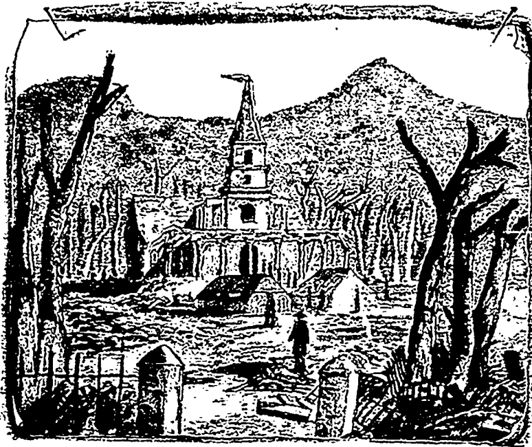
MAURITIUS CATHEDRAL AFTER THE HURRICANE.
