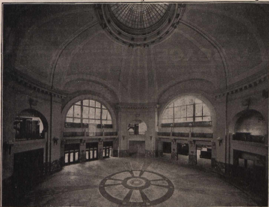
Fort Garry Union Station, Winnipeg. Ticket Lobby.
