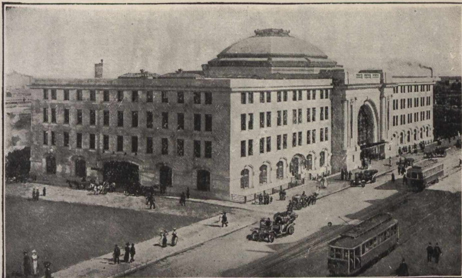
Fort Garry Union Station, Winnipeg.
