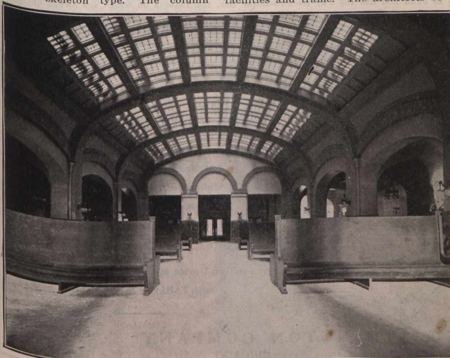
Fort Garry Union Station, Winnipeg. Waiting Room.
