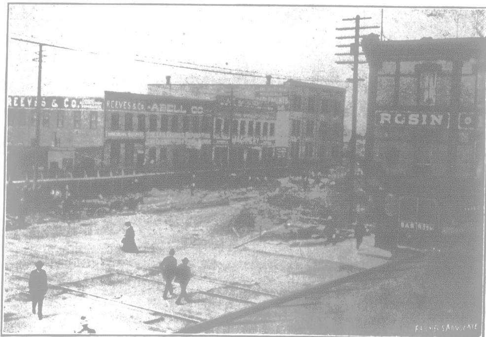
At Work on the Main St. Subway, Winnipeg.
