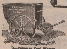
4—Furnace Coal Wagon
