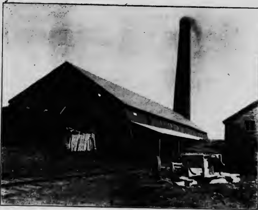
Fig. 38.—16-chambered continuous down-draft kiln, capacity 340,000 brick; Port Credit Brick Co.
