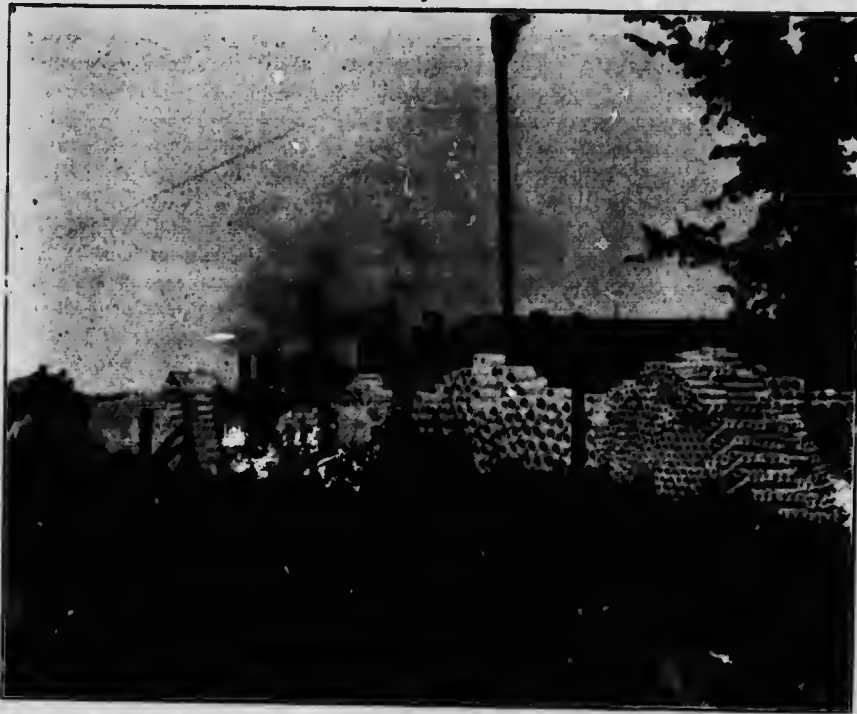
Fig. 50.—Beaverton Brick and Tile Co's yard, Beaverton. Note round down-draft kilns burning coal.
