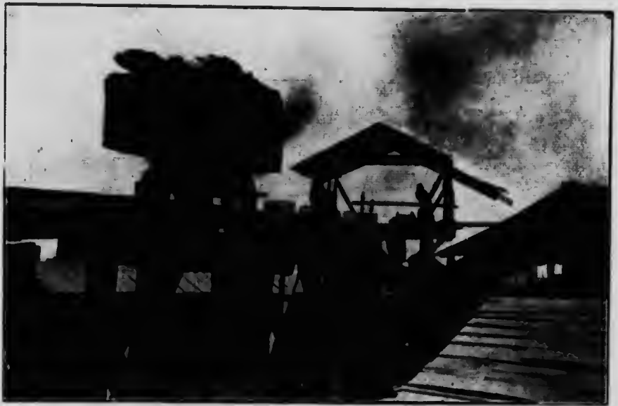
Fig. 27.—Clay brought over the tops of the hacks by clay cars and cable, F. Entricken's yard, Stratford.
