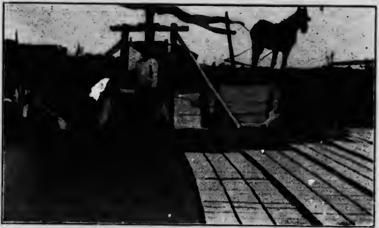
Fig. 30.—Slop-brick plant in operation, Crediton. The brick are dried in the open yard as shown in the photo.
