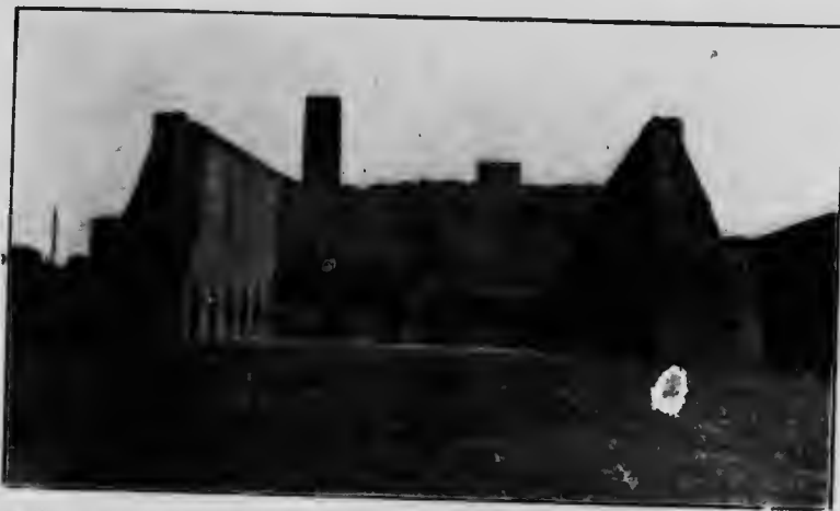
Fig. 35.—Permanent walled up-draft kiln, capacity 250,000 brick; London Builders' Supply Co., London.
