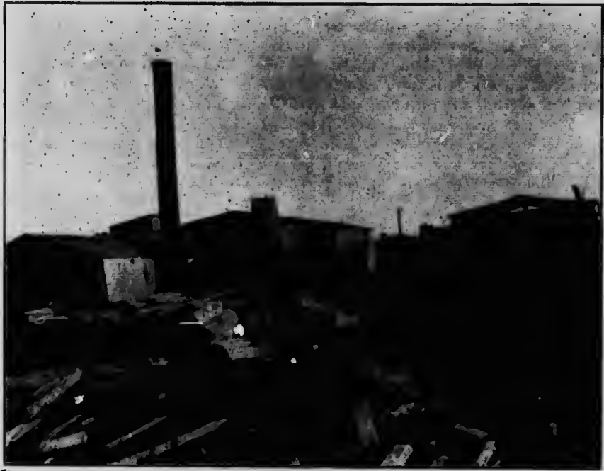
Fig. 56.—Merkley Bros' yard, Casselman; showing the scoved kilns and drier.
