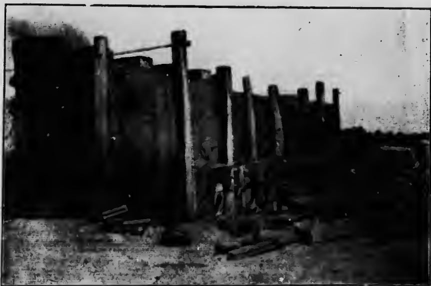
Fig. 37.—A rectangular down-draft kiln, capacity about 120,000 brick.
