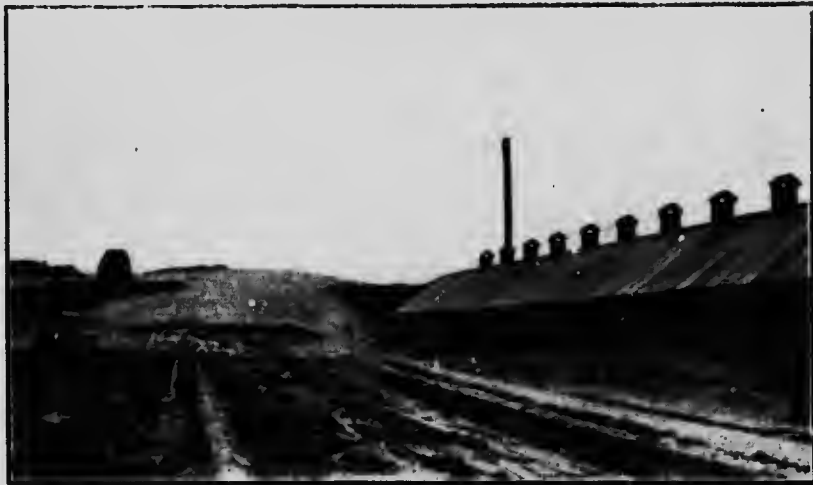
Fig. 59.—A former "hack" yard replaced by a Bechtel Carless dryer; Branford Brick Co's yard.
