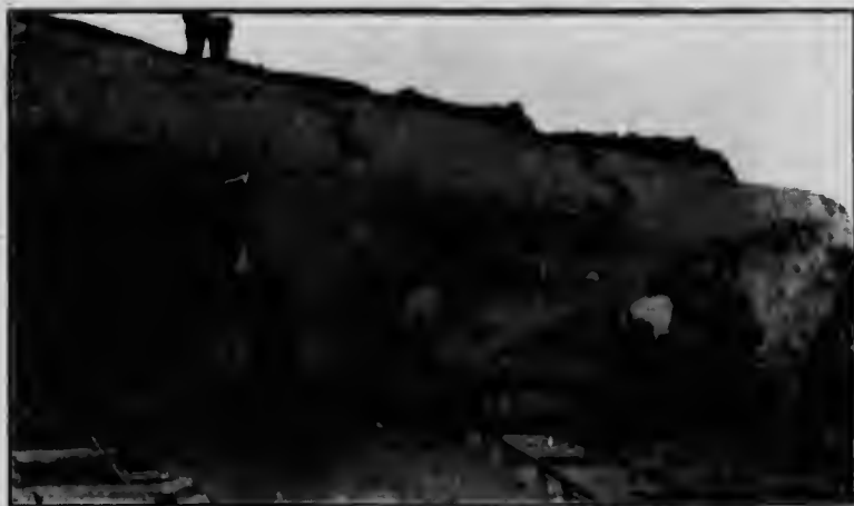
Fig. 22.—Section of lacustrine clay at Builders' Supply Co's plant, London; four feet of gravel is removed from top for road purposes. The light band is a very strong clay.
