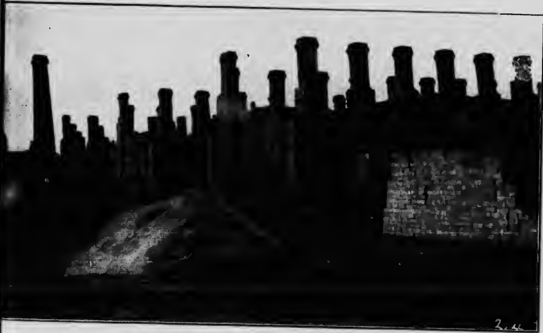
Fig. 65.—Rectangular down-draft kilns for burning paving brick ; Ontario Paving Brick Company.
