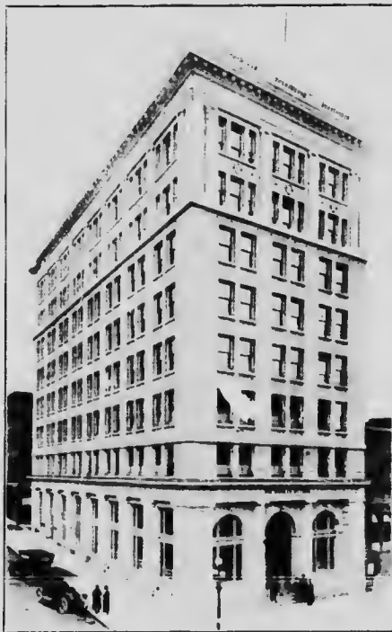
Richards Street now nearly completed.
