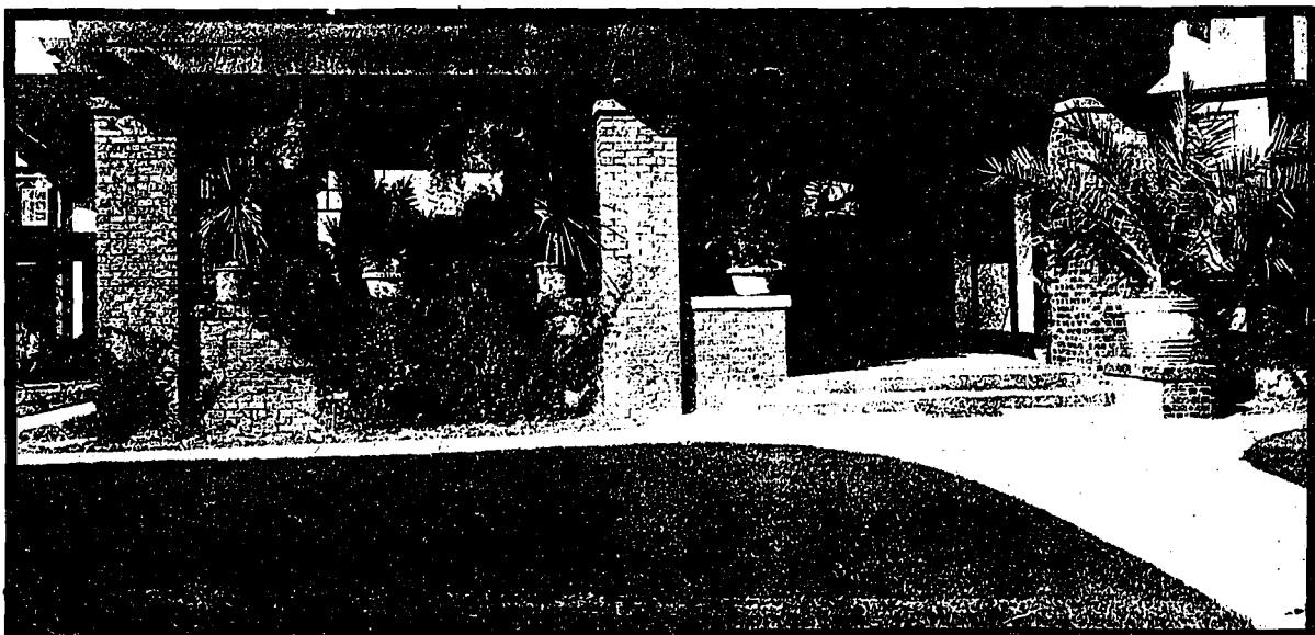
Detail of Covered Porch, Residence of Mrs. H. B. Kling. R. Mackay Fripp, Architect.
