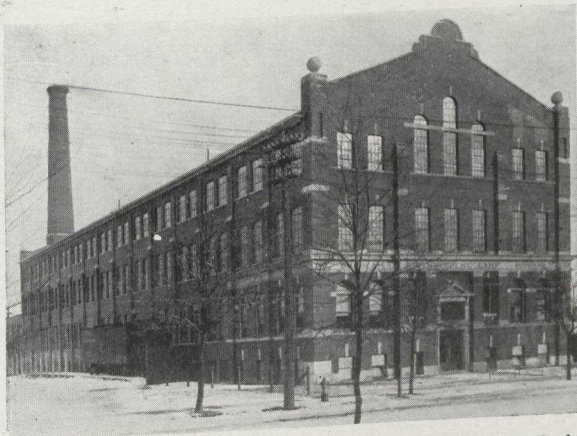
Sunbeam Incandescent Lamp Co.'s Building, Dufferin Street, Toronto. F. Herbert, Architect. W. J. McGuire, Limited, Plumbers.
