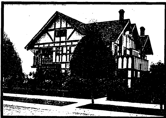
Residence of Mrs. H. B. Kling, as It is Seen from the Roadway. R. Mackay Fripp, Architect.
