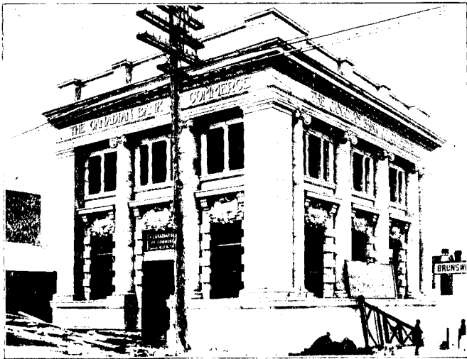
Canadian Bank of Commerce, Brandon. Darling & Pearson, Architects.
