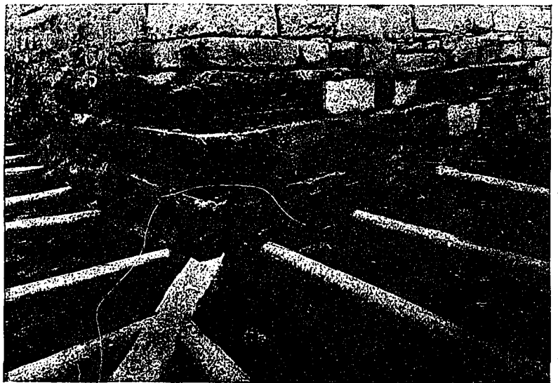
Widening the Foundation, Showing the Old Masonry Work and the Piling for the New Section.
