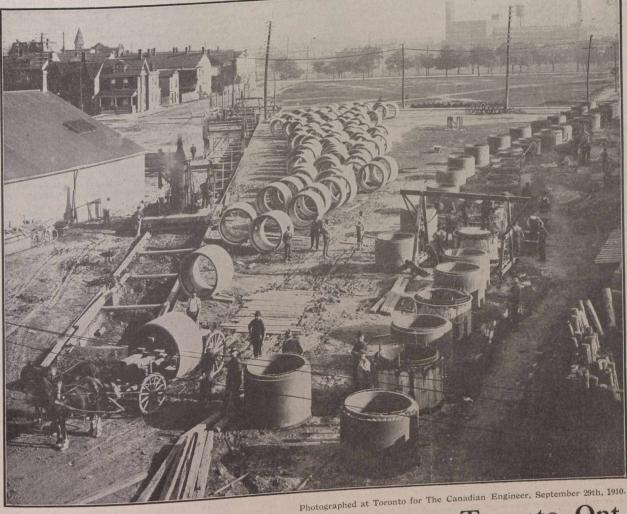
60-inch Pipe for Intercepting Sewer, Toronto, Ont. LOCK JOINT PIPE CO. 167 BROADWAY - NEW YORK CITY Write for Illustrated Catalog.
