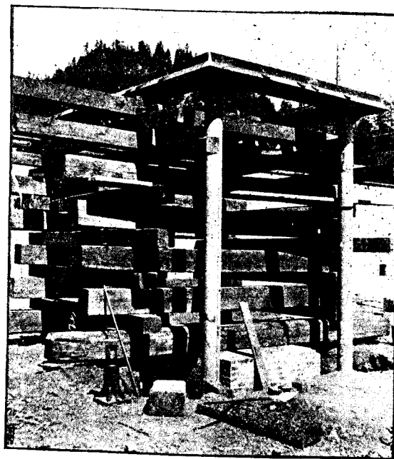
The Furnace in Building.
