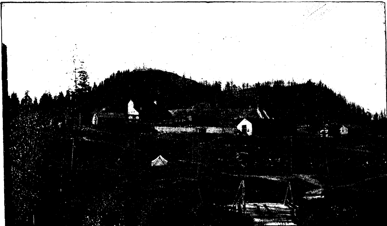
General View of Smelter Site Looking North from Anaconda.
