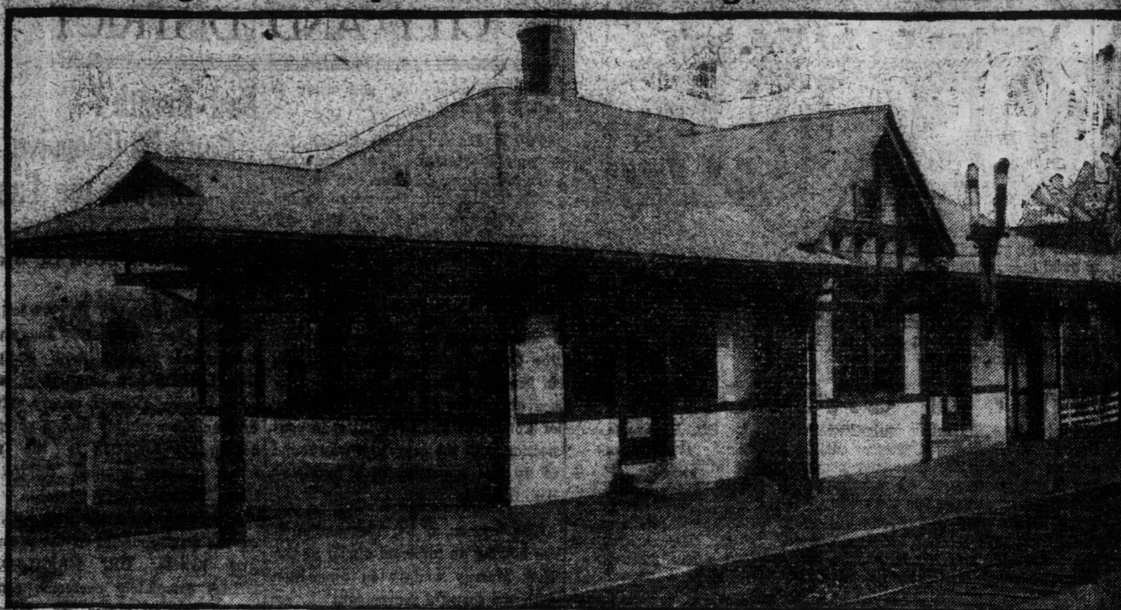
The new Dominion Atlantic Railway Passenger Station at Bridgetown.
