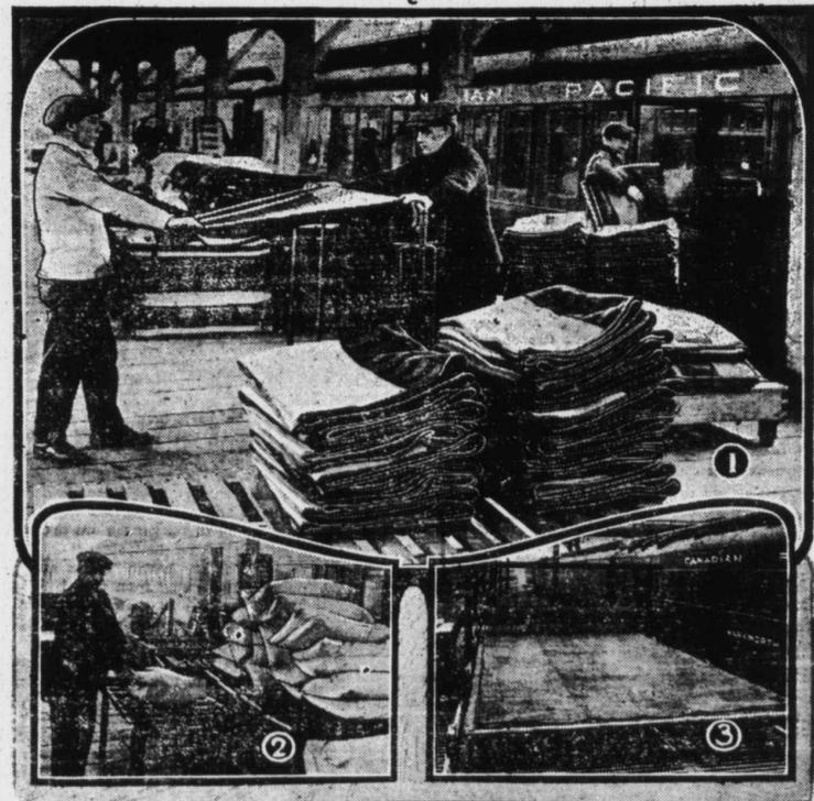
1. Packing away the rugs after having had their turn on the vacuum. 2. Cleaning the pillows on the vacuum cleaner invented by Canadian Pacific employees. 3. The train carpet beater in action. Straps attached to the roller quickly loosen all dust.
