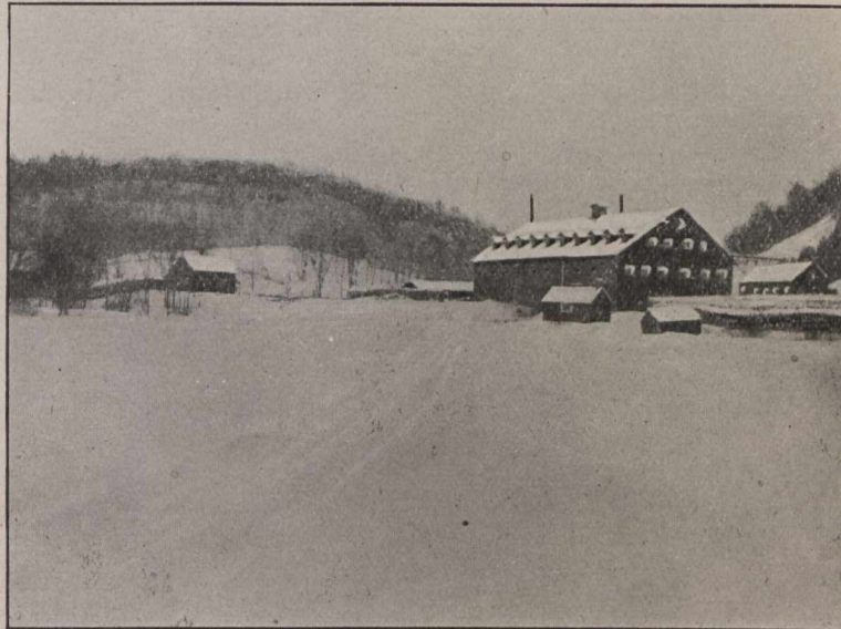
Mill of the Buckingham Graphite Co.—Reconstructed by Mr. H. P. H. Brumell.
