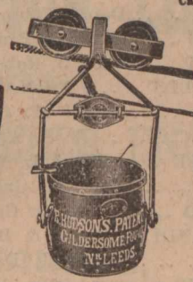
61—Rope Bucket, with R. H.'s Patent Catch for Wire Rope Progress
