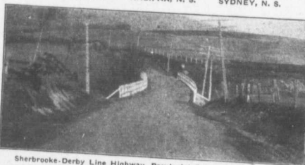
Sherbrooke-Derby Line Highway, Provincial Government of Quebec. Constructed with "Tarvia-X" in 1915.
