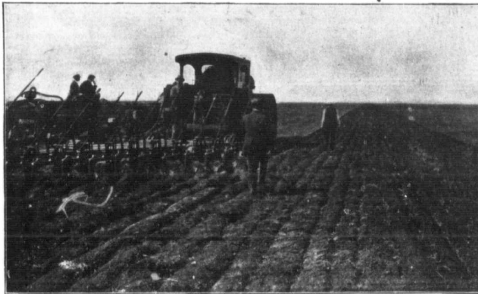
The Avery 30 H.P. Double Under-mounted Steam Tractor (Winner of Gold Medal Steam Class, 1911 Motor Competition), doing its Gold Medal Plowing Stunt with a 10 bottom 14 inch Cockshutt Engine Gang
