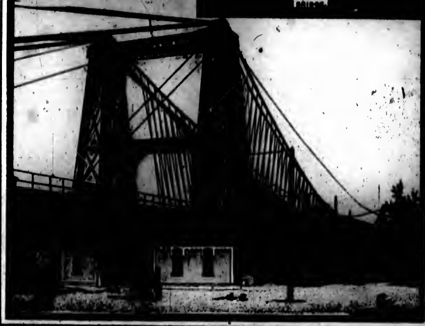
OLD RAILWAY SUSPENSION BRIDGE.
