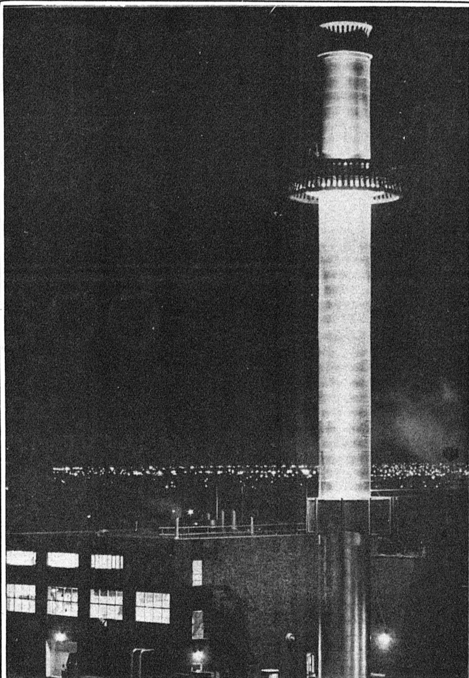
$733,000 170-foot addition to the university power plant.
