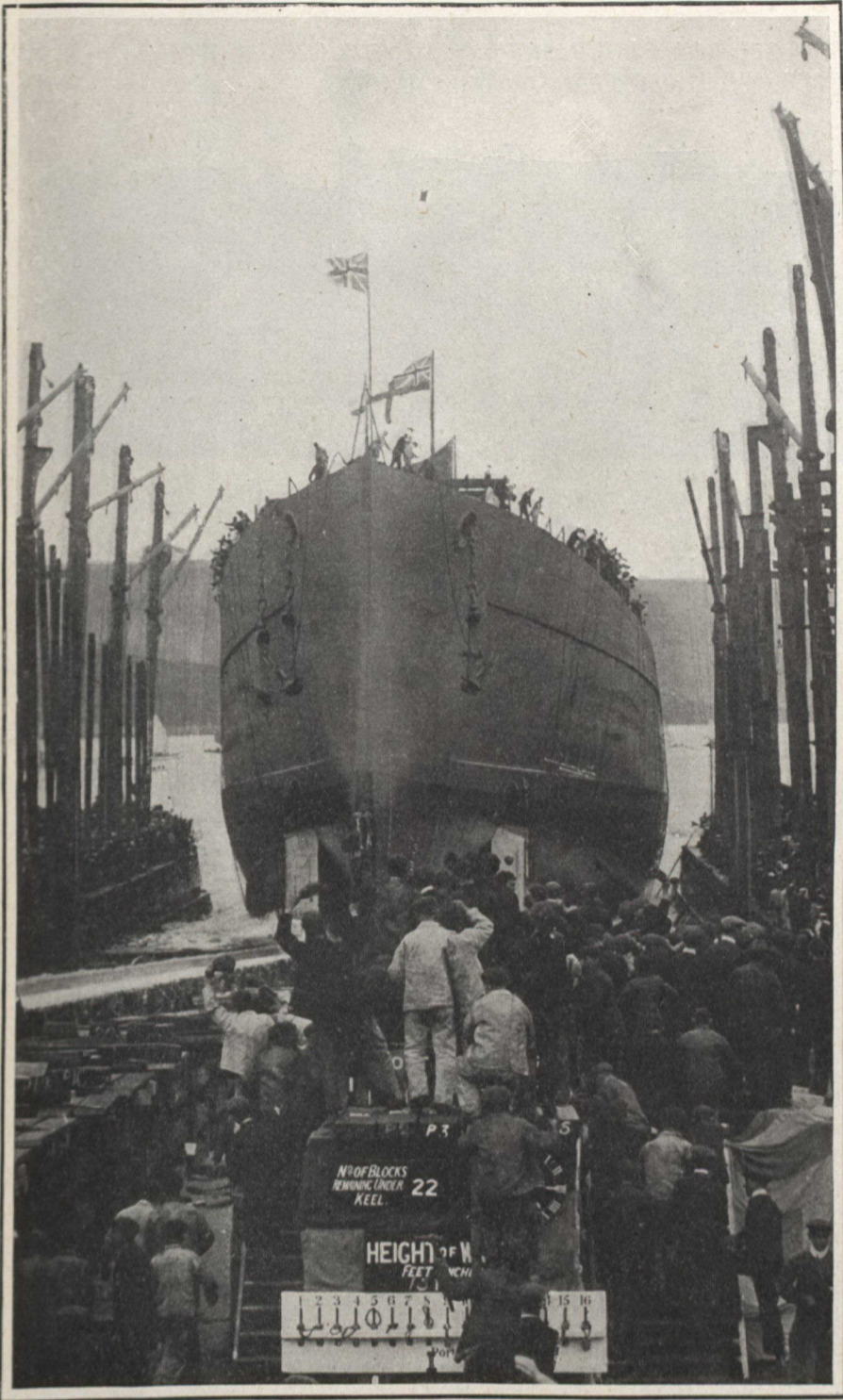
The Battleship-Cruiser "Lion"—the mystery ship of the British Navy was launched recently, at Devonport. The "Lion" is more powerful than the most powerful Dreadnought. When completed it will displace 26,360 tons, nearly half as large again as the original Dreadnought which displaces only 17,900 tons. Her total cost will be over ten million dollars.
