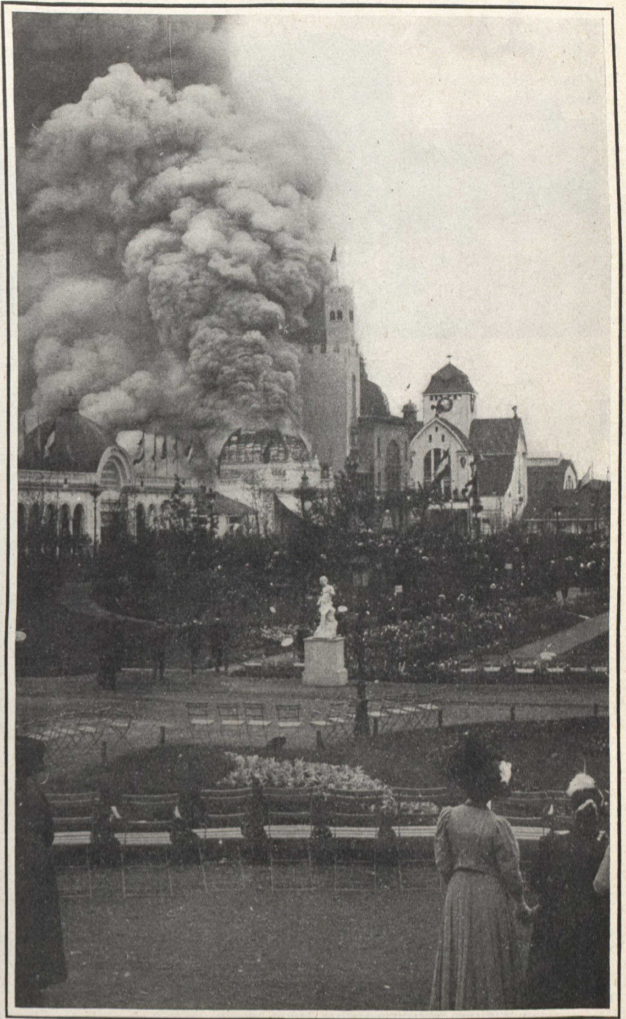
The Fire which destroyed a portion of the International Exposition at Brussels, Belgium. This picture shows the German Pavilion and the Cafe Metropole in course of destruction. Unlike the buildings at the Toronto Exhibition, which are practically fire-proof, these buildings were of the flimsy construction usual with temporary Exhibition Buildings.
