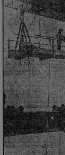
This view shows men at work on extremity of the great span, driving the main top center pin, 375 feet above the water.
