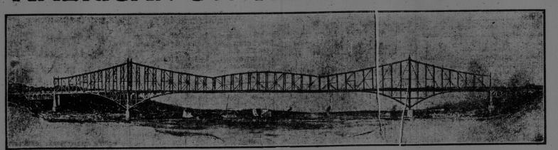
LOUISBURG, C. B., Aug. 20.—Rival- The bridge as it will appear when completed. Total length 3,600 feet, centre span 1,800 feet, Floor is 150 feet above low water. Towers 360 feet above.
