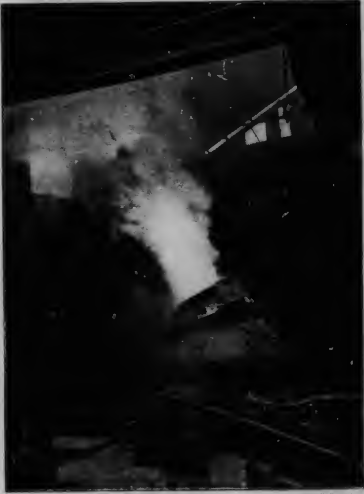
Basic Bessemer converter during blow, at works of Dominion Iron and Steel Co., Sydney, C.B.
