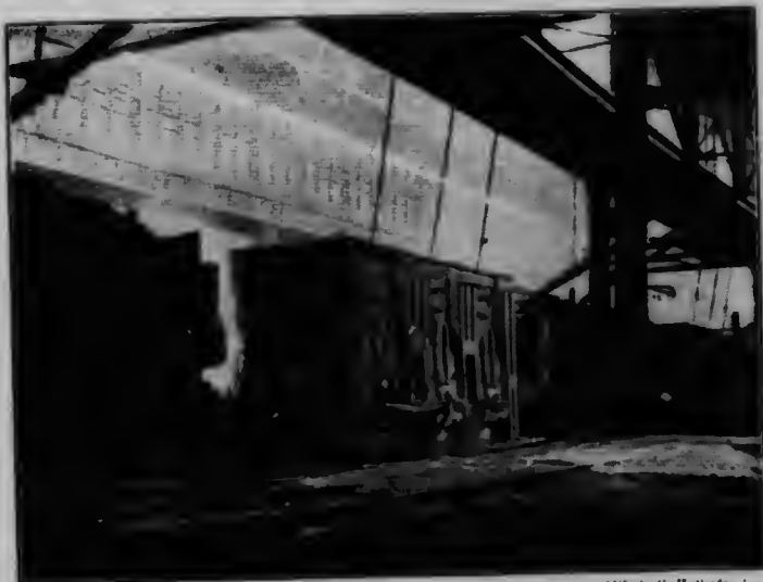
Basic open-hearth furnace—charging side—at Dominion Iron and Steel Company's works, Sydney, C.B.
