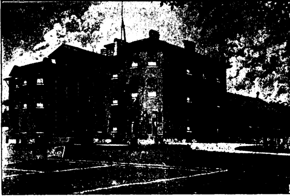
SOUTH AND EAST FRONTS, SHOWING CHAPEL
