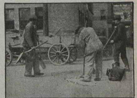
Screenings are scattered over the seal-coat and the patch is again tamped.
