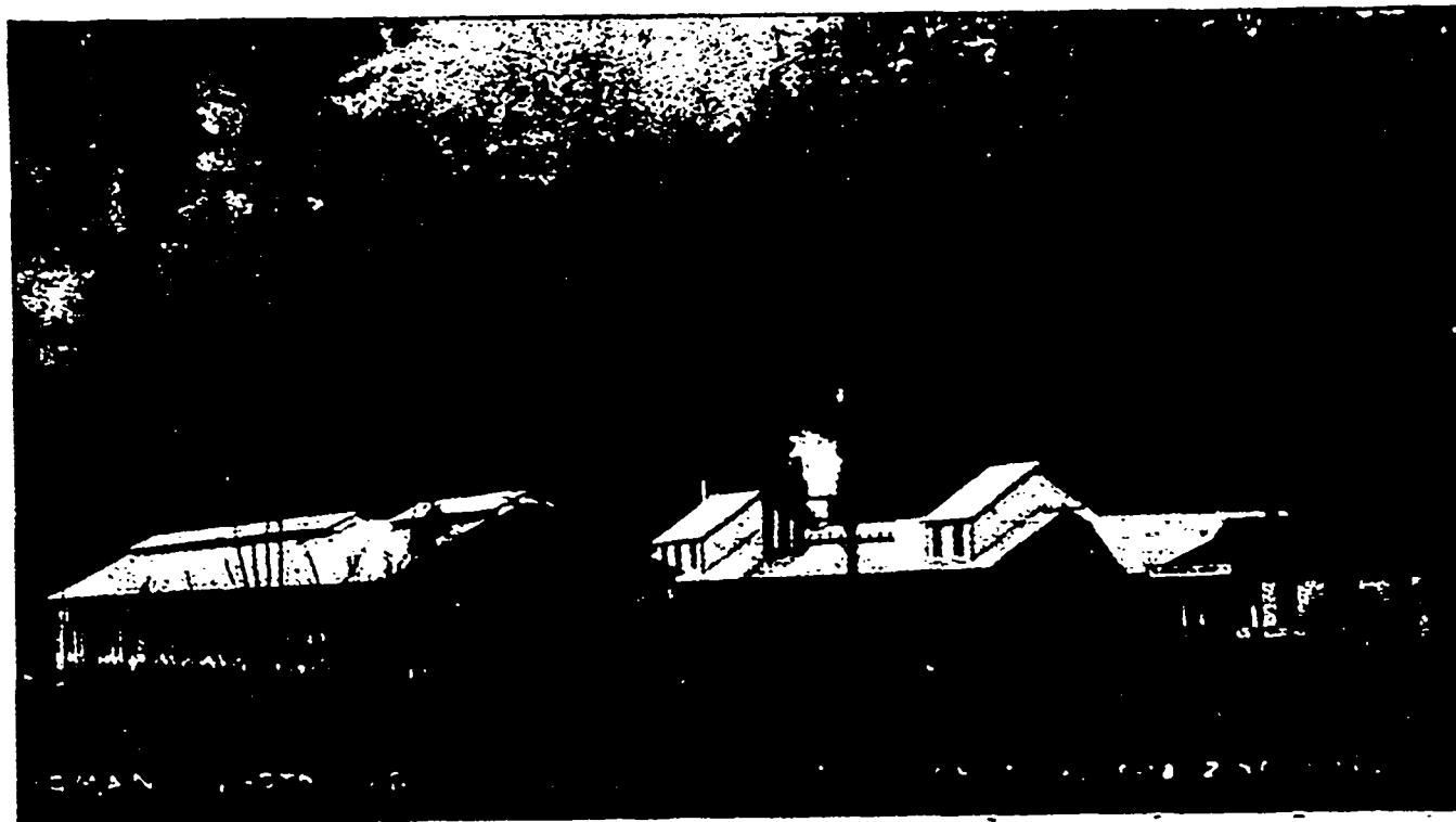
Canadian Metal Co's Zinc Smelter, at Frank, South-west Alberta. Built and equipped in 1905.
