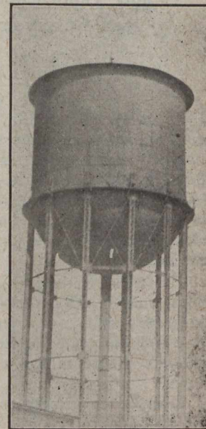
One of the Largest Elevated Steel Water Tanks in Canada
