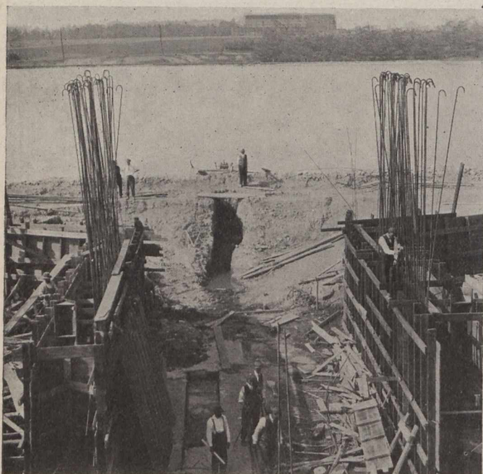
Fig. 11.—Reinforcing Work for the Supply Weir. Section 4A.
