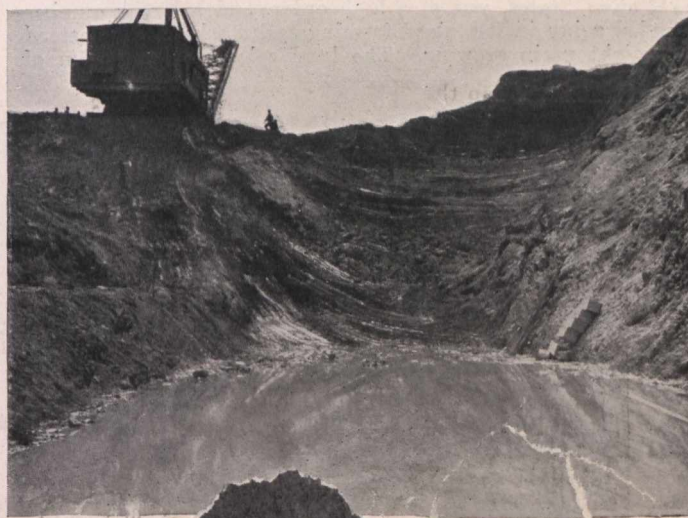
A BUSH COUNTRY. EXCAVATION WORK.
