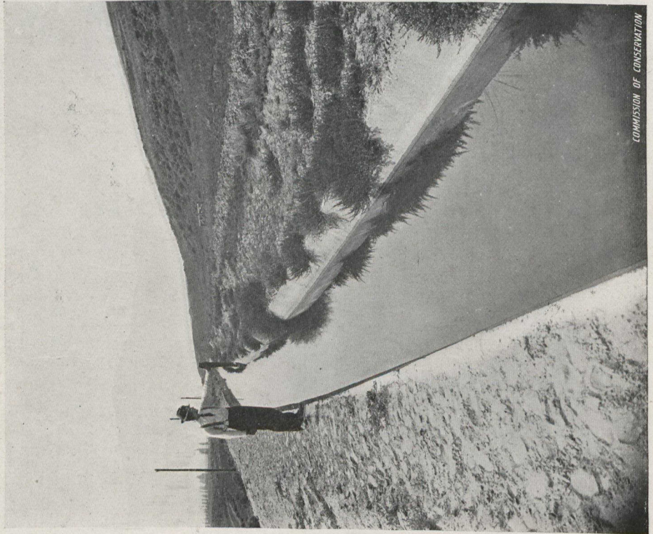
How water is sometimes carried in Western Canada for small power and irrigation purposes. The first picture shows a ditch lined with concrete; the second, a wooden flume skirting a mountain side.
