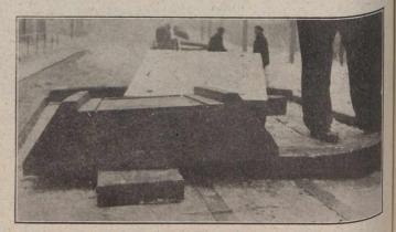
Fig. 5.—Cast Steel Bed Plate, Showing Inset for Bronze Plate.
