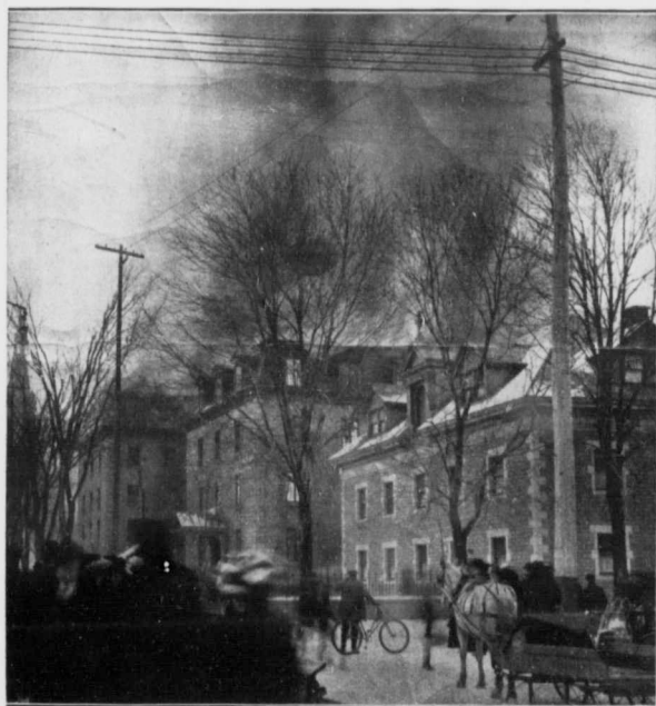
Scene during the Fire.—Sisters' House in foreground was saved.
