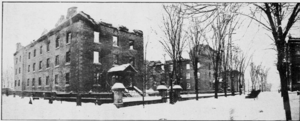
RUINS AFTER THE FIRE. View from the north east angle.
