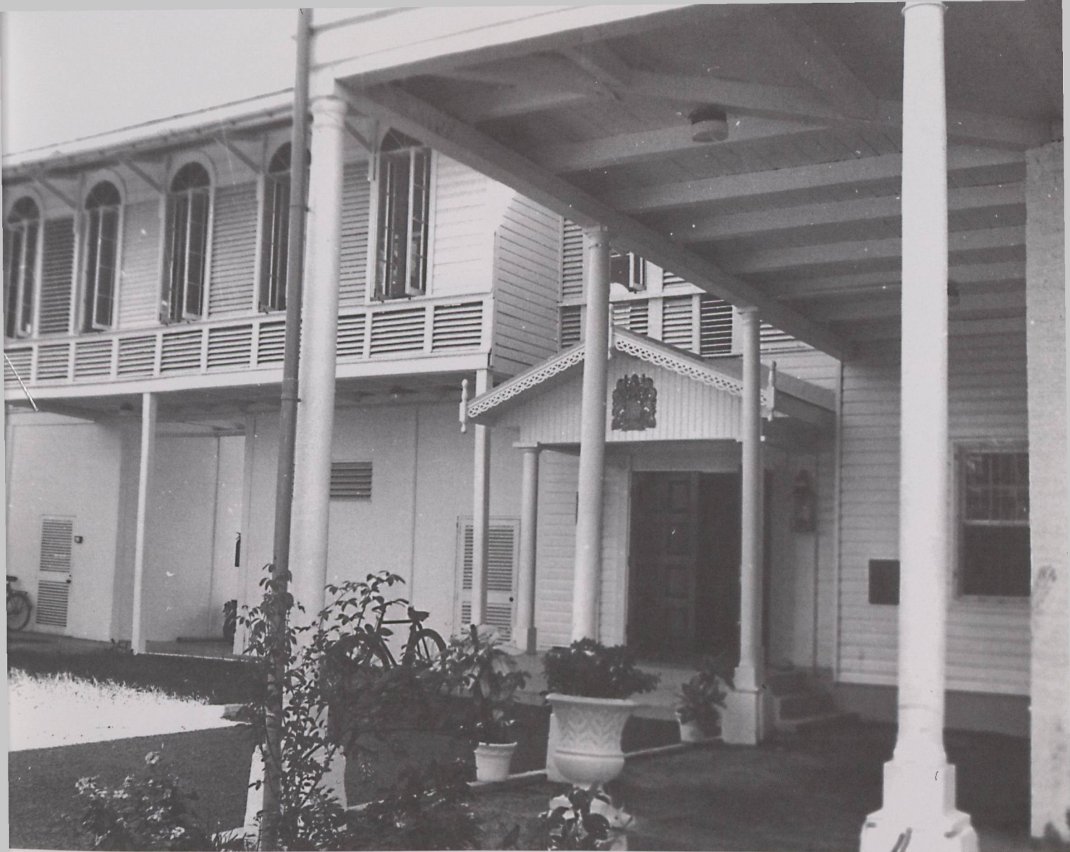
MAIN ENTRANCE of the High Commission.
