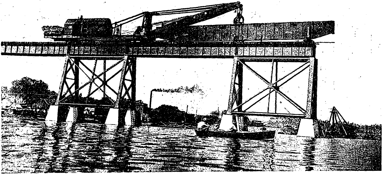
NO. I.—FASTENING THE TACKLE TO LIFT THE 114-FOOT GIRDER.
