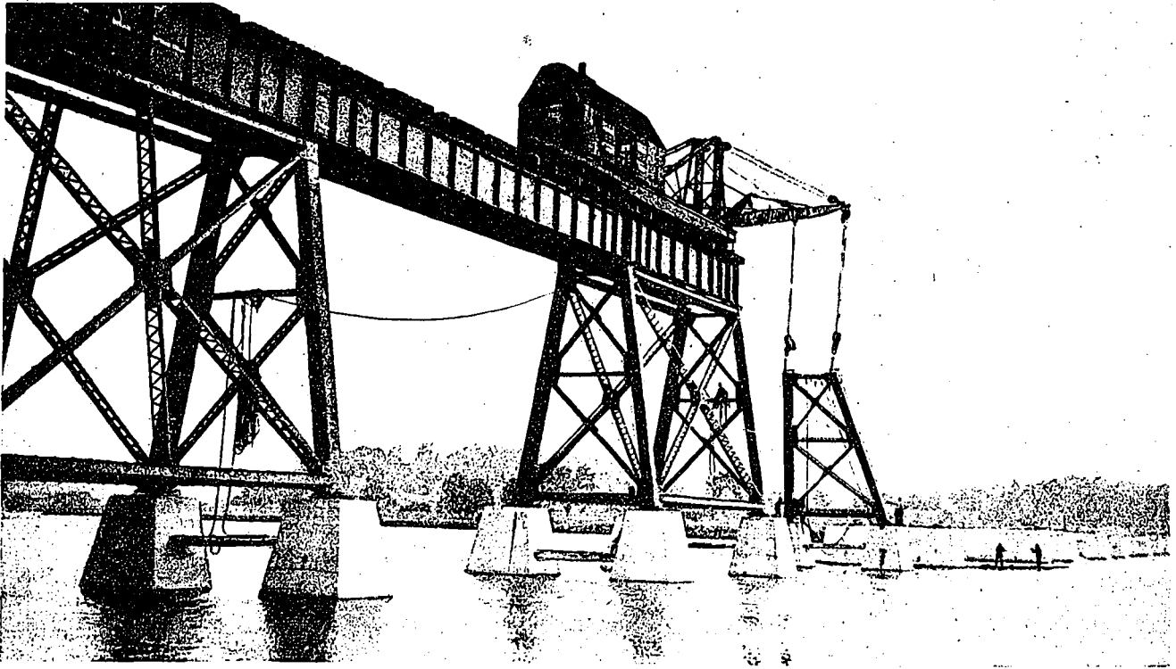
NO. V.—UP-ENDING A BENT BY MEANS OF DERRICK CAR.
